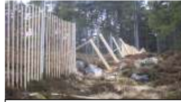
Deer fence marked with wooden droppers
